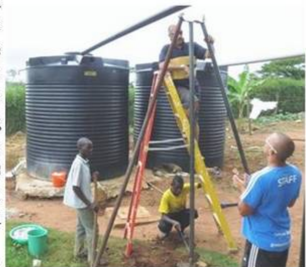
Repairing the water tanks
